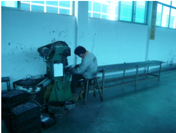
Cutting steel rods
